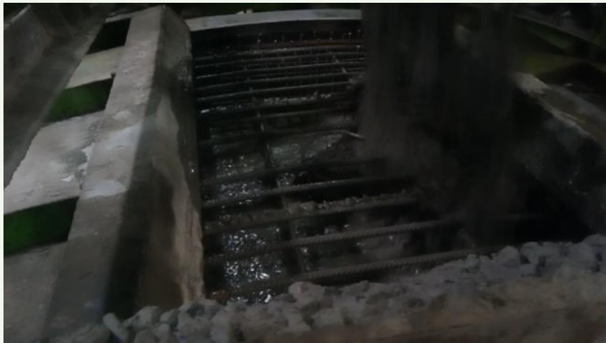
Pouring of fresh concrete with POLYPLAST PC type S Good flow of concrete
